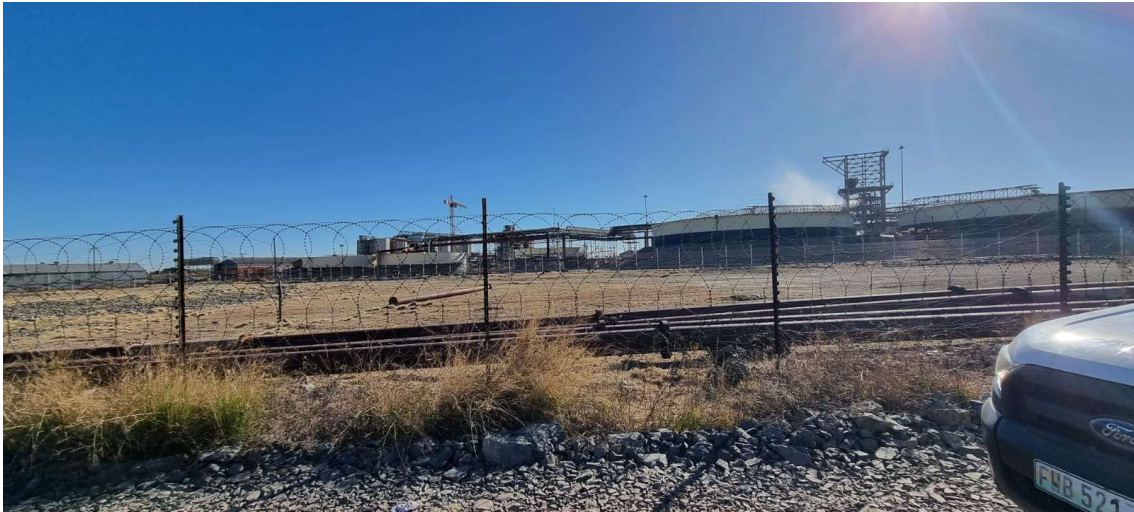
East view of the Saaipiaas Gold Plant.
