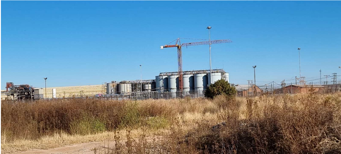
North view of the Saaipiaas Gold Plant.
