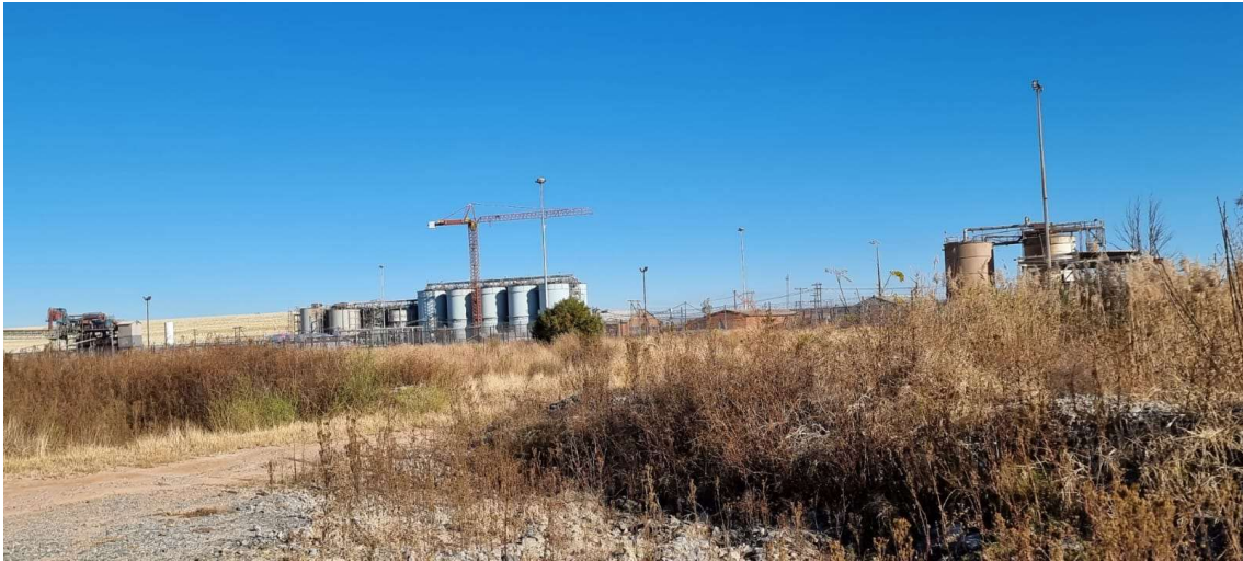
North view of the Saaiploas Gold Plant.
