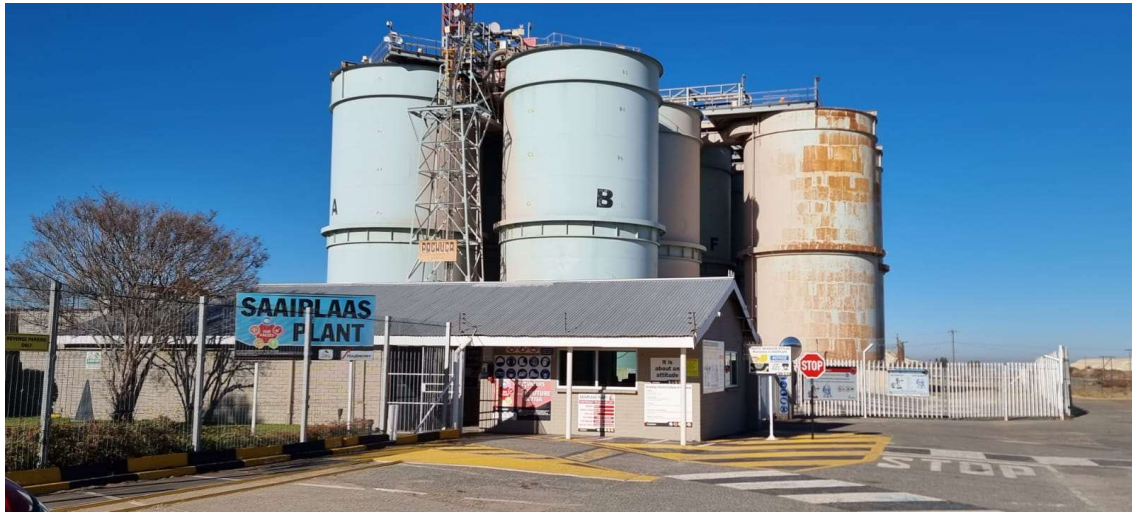
South-west view of the Saaiplaas Gold Plant.
