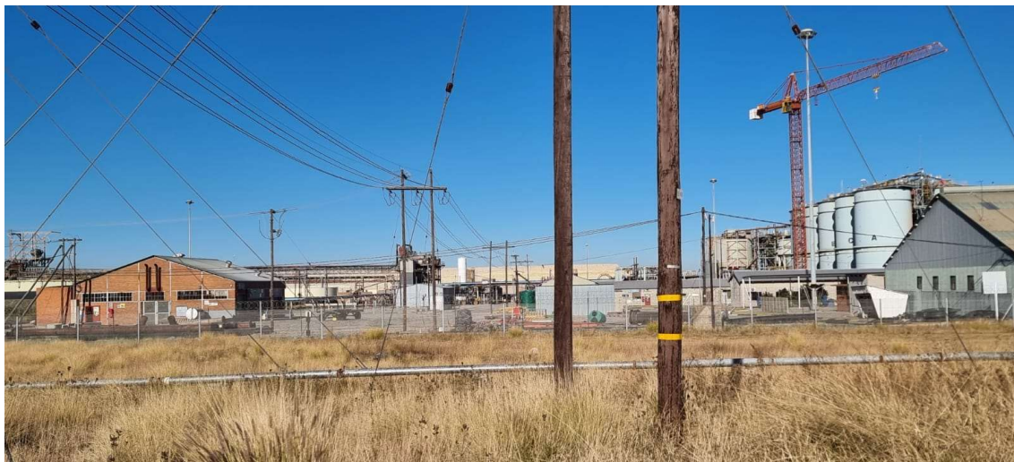
West view of the Saaiplaas Gold Plant.
