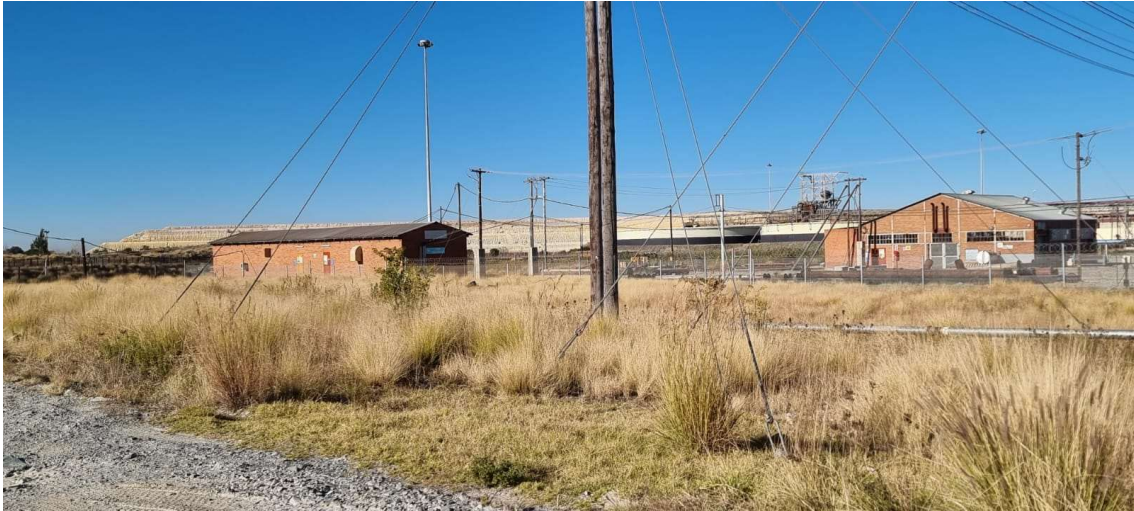
North-west view of the Saaiploas Gold Plant.
